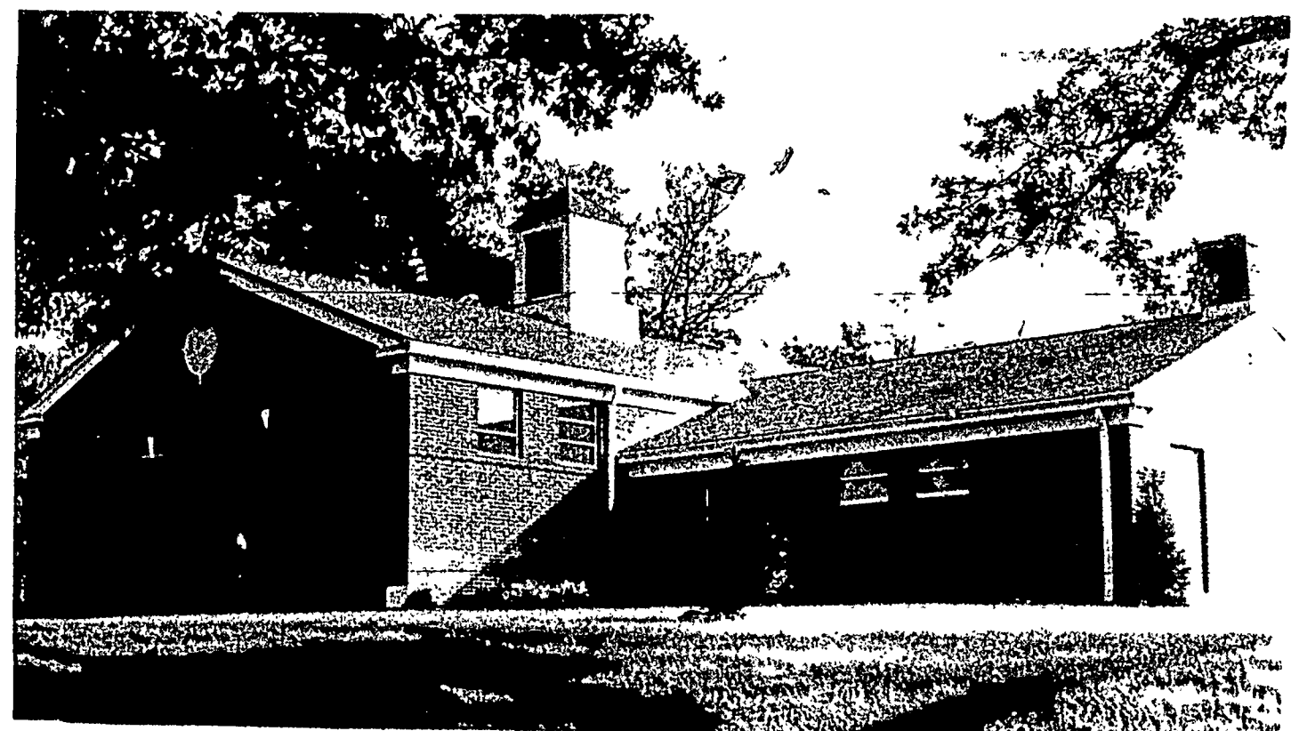
New North Salem Firehouse
